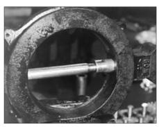
**Figure 6 -** Shaft bushing flush with the flow path surface.
